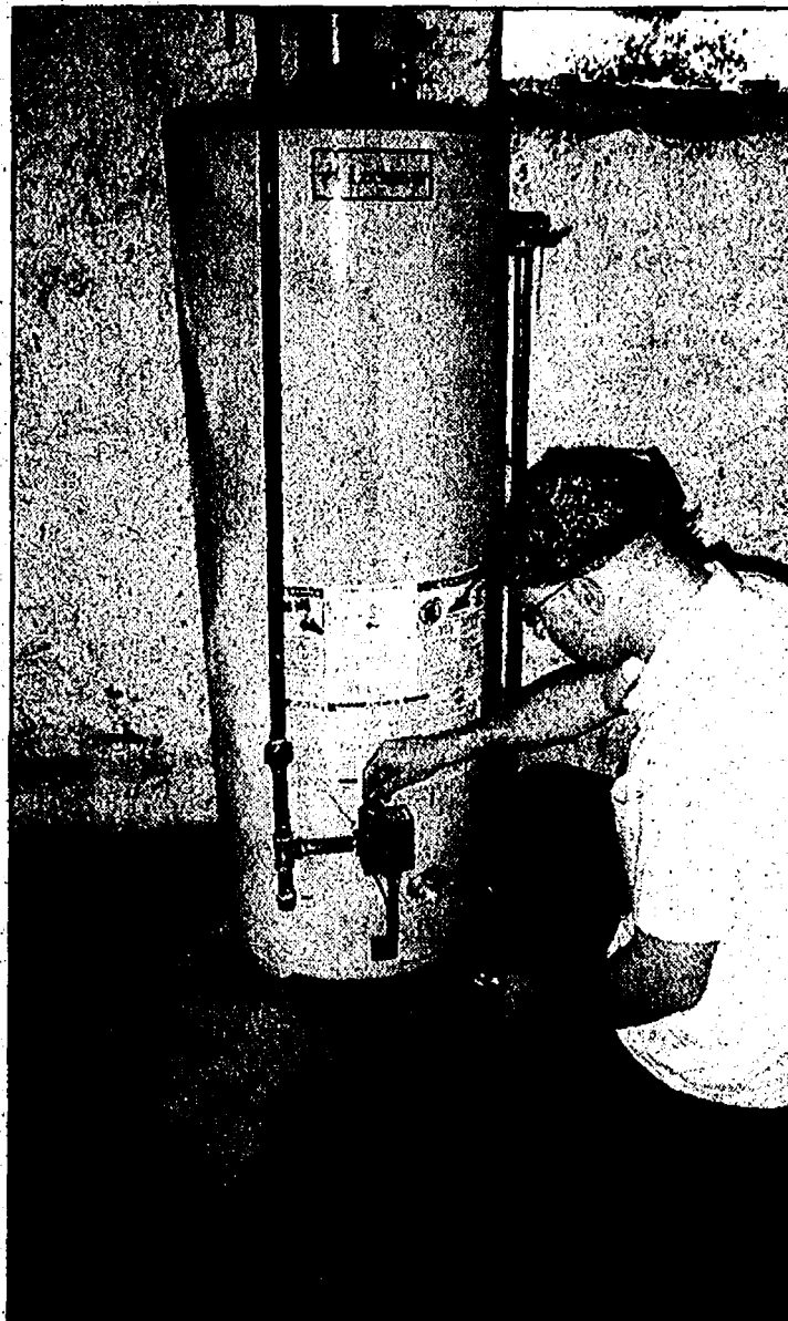
Frank Currie of Elemental Habitats adjusts the pilot of a hot water heater in preparation to test a home for energy efficiency.
